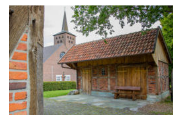
St. Nikolaus Diestedde, Backhaus, Remise
