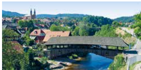
Holzbrücke in Forbach ▶
